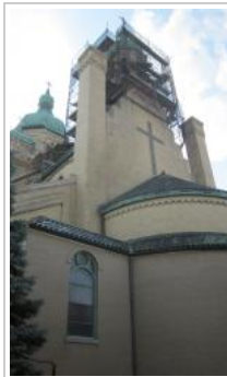
A southeast view of the structure
